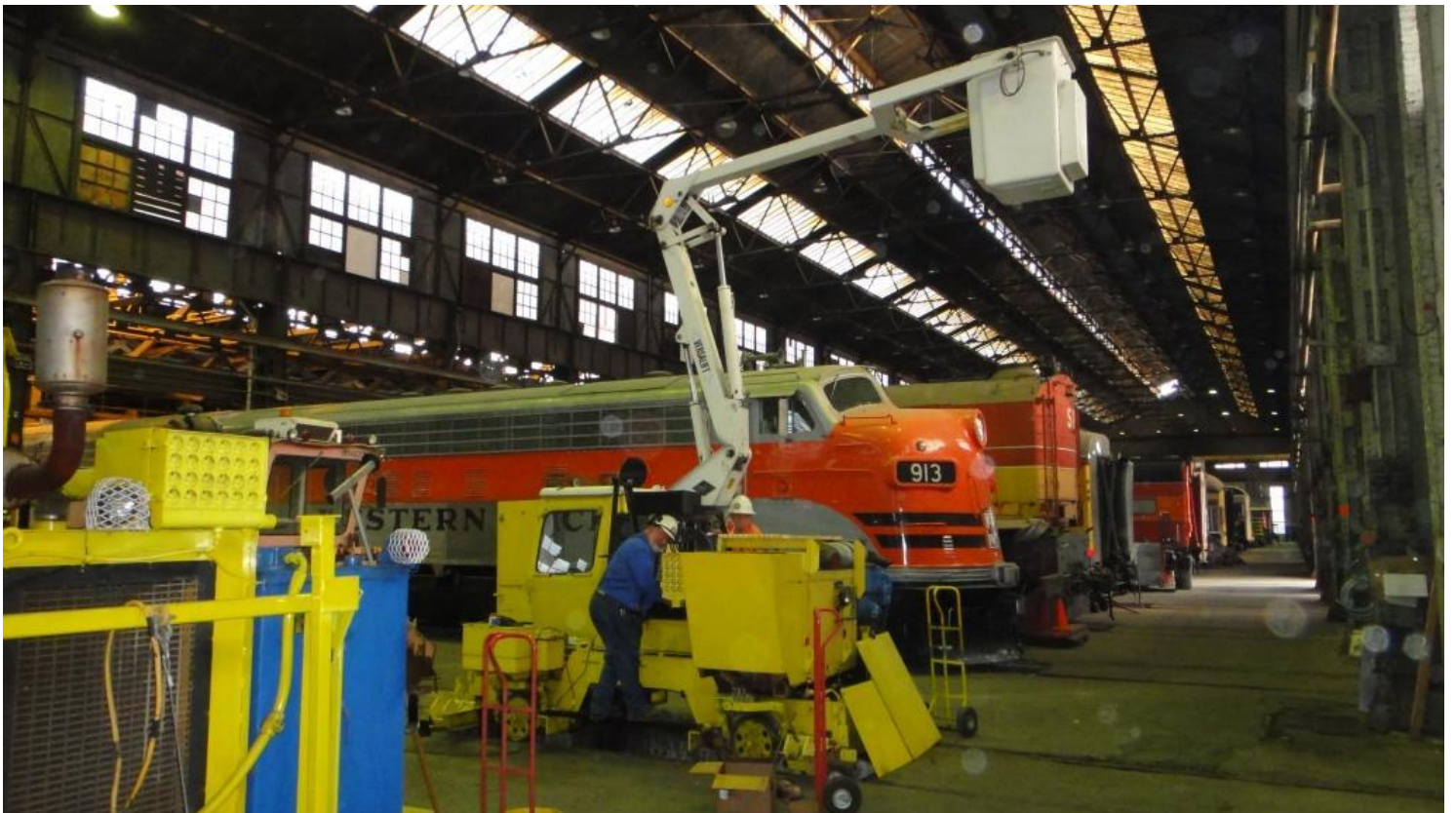
Success! The new swivel-gear works! Frank and Mike H. deploy the bucket and test the repaired system
