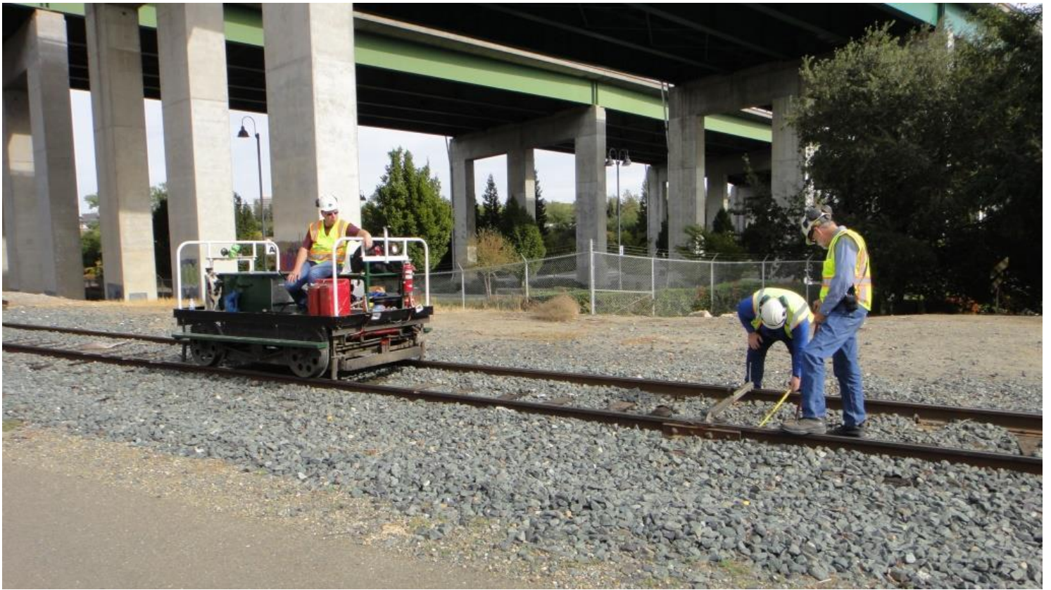
Trusty Team Track Inspection Ed, Frank, and Alan, were out on the line checking gauge in an area with a couple of skewed ties while marking bad ties for the big tie replacement push
