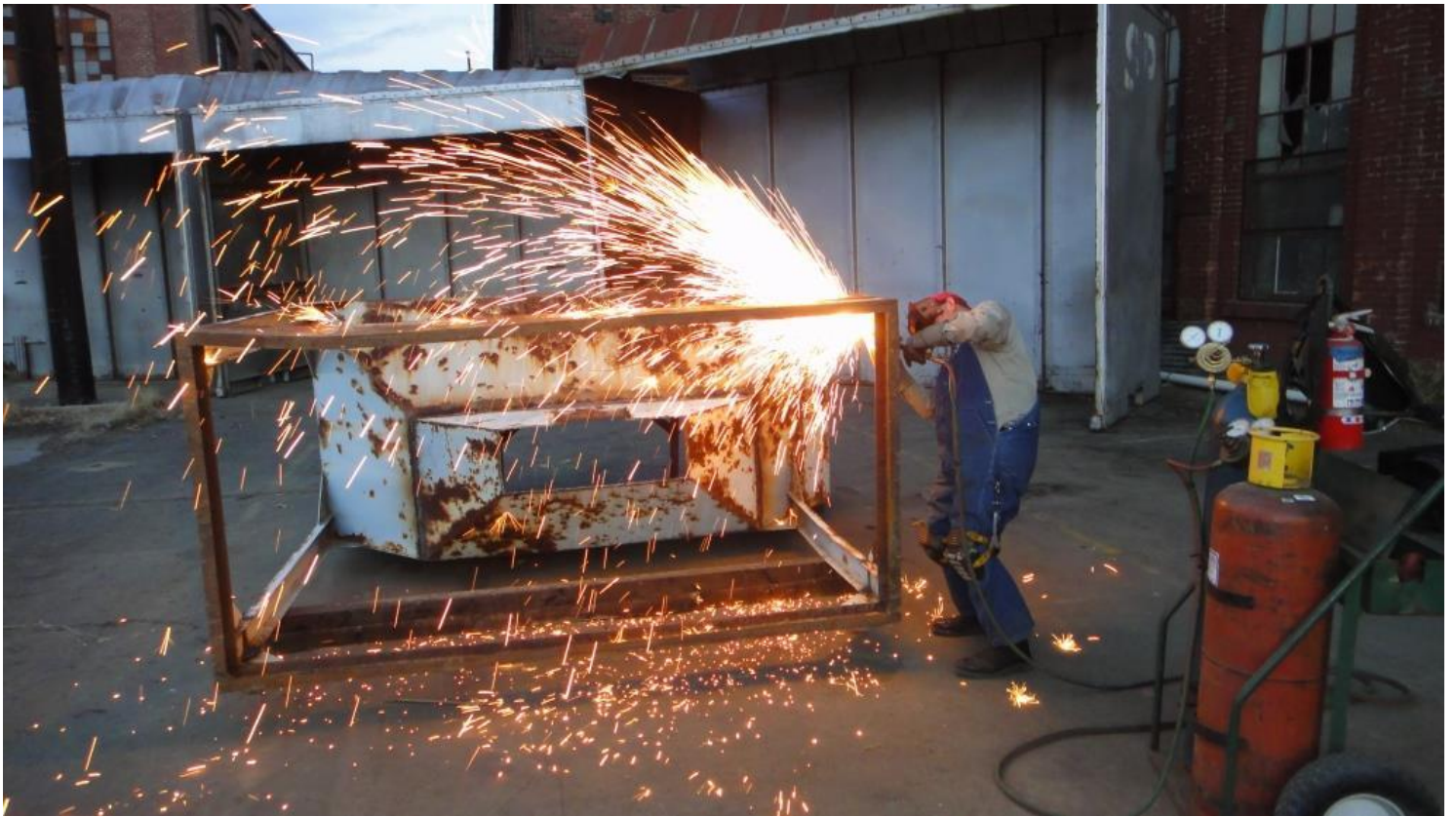
Is it the Fourth of July? No, it's Cliff cutting down the legs of the new ballast hopper preparing it for its rail wheels
